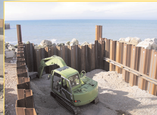
Work starts on the new West Pier
