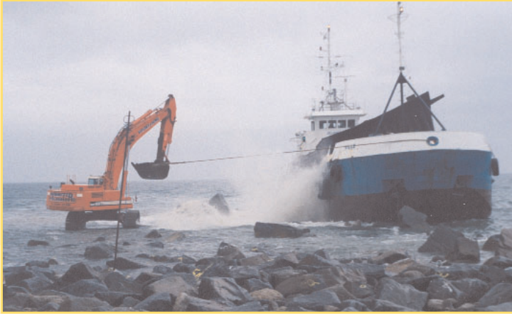
Rock armour is delivered by sea
